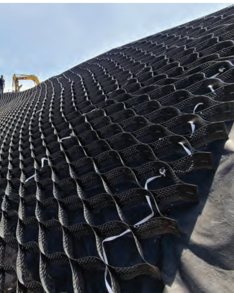
After River Walk Installation w/ Presto Geoweb Support
