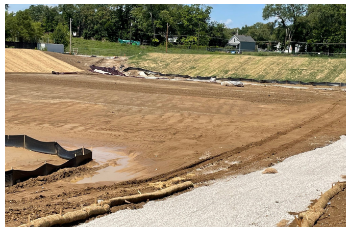
The sides of the basin are covered with erosion control blankets to protect the grass seed as the vegetation is established. The bottom of the basin will be covered in ECBs and vegetated as well.
