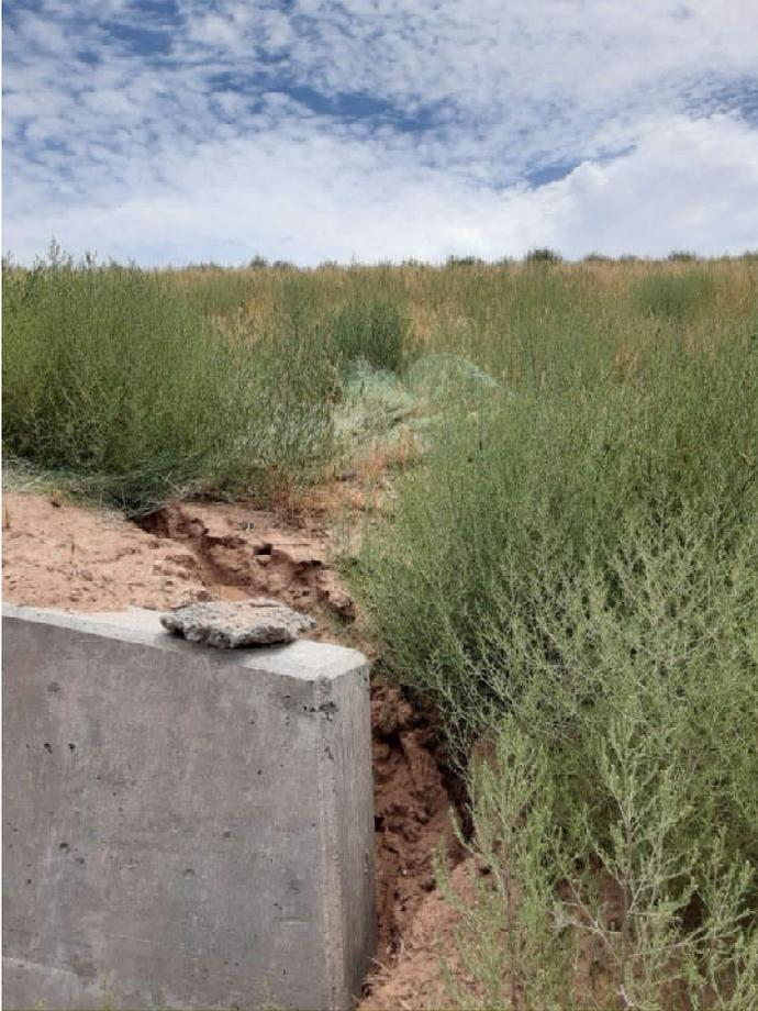
Plastic netting that has grown up with the tumble weeds causing the washout behind the box wingwall
