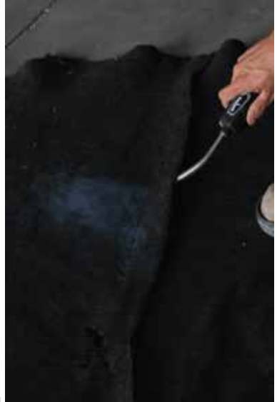
Figure 29: Geotextile being melted together with a torch.
