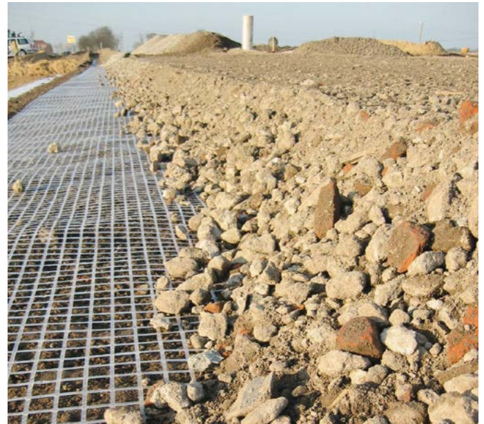
Fig. 19 Crushed base course material over Naue Secugrid® for base stabilisation in access roads
