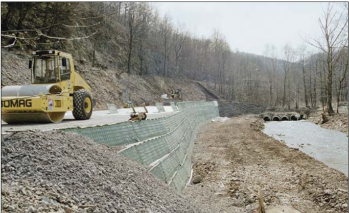
Railroad slope stabilisation
