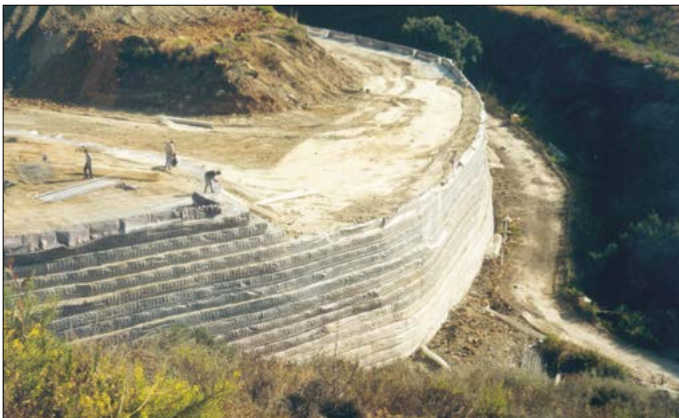
Mechanically stabilised earth (MSE) wall construction
