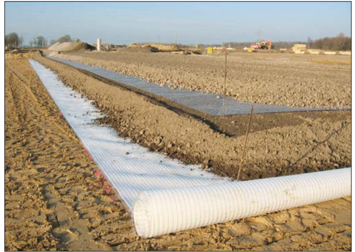
Fig. 8 Base course reinforcement on a very soft subsoil with Naue Combigrig® (bottom) and Naue Secugrid®
