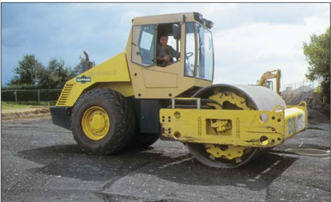
Compaction of aggregate on top of Secugrid®
