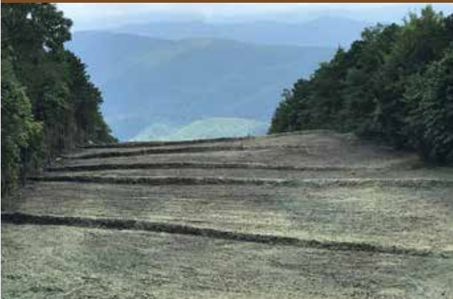
Energy / Pipeline Restoration
